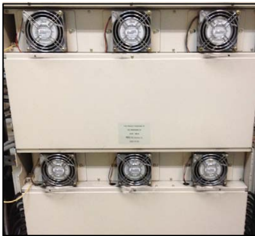
NEC FD-31201A / FD-32401A LINE TERMINATING MULTIPLEXER UNIT w/ DEFECTIVE FANS
