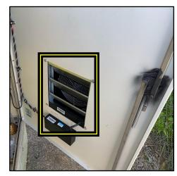
HEAT EXCHANGER MOUNTED IN THE DOOR
