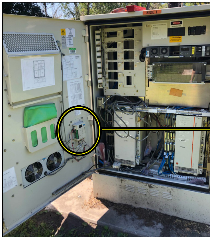
INSIDE VIEW OF MESA 384 CABINET (EXISTING ECU IS MOUNTED ON THE CABINET DOOR)
