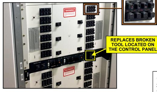
PN # T-5ESSPCT **5ESS** Pre-Charge Tool (control panel pre-charge tool replacement)
