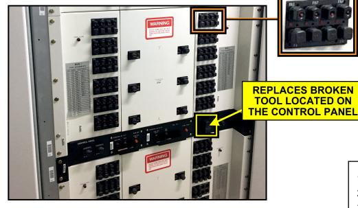
PN # T-5ESSPCT 5ESS Pre-Charge Tool (control panel pre-charge
