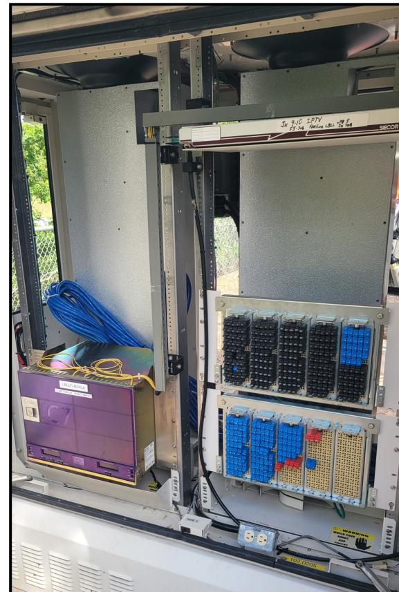
The **TFC-ALMSTRP-01** provides a hardened termination for added additional intrusion alarms such as "door open", fan failed, thermal sensors, or any other external wired alarm when the original DISC\*S, AFC, UMC, ADTRAN TA5K, TA3K has been removed from service.
